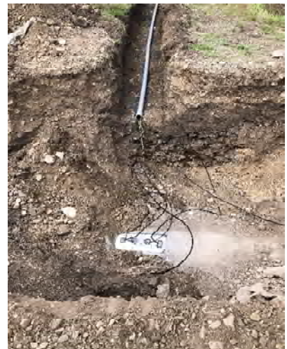
Cables cad welded to the 42-inch pipeline
