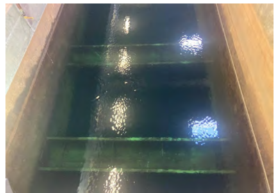
Low turbidity influent water to north filters showing the high efficiency of the recently installed plate settler technology in Basins 3-6
