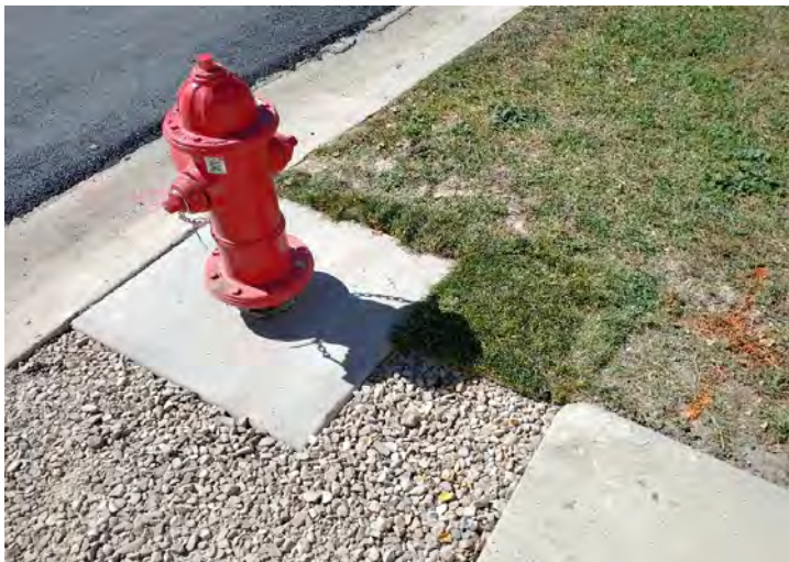
Newly installed fire hydrant with pad and restored landscape
