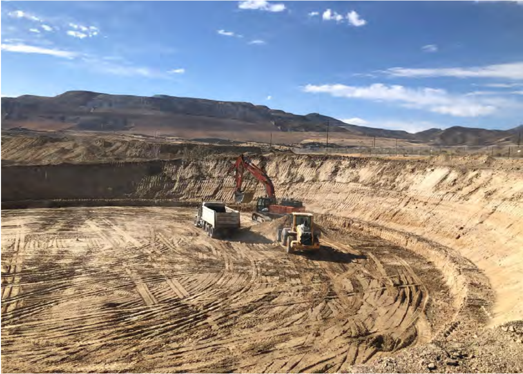
Excavation of subgrade for the east tank
