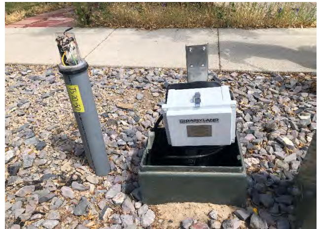
DC blocker and test station
