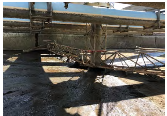
Circular clarifier mechanism to be removed as part of this project
