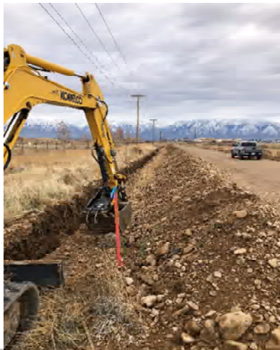
Excavation to install cable
