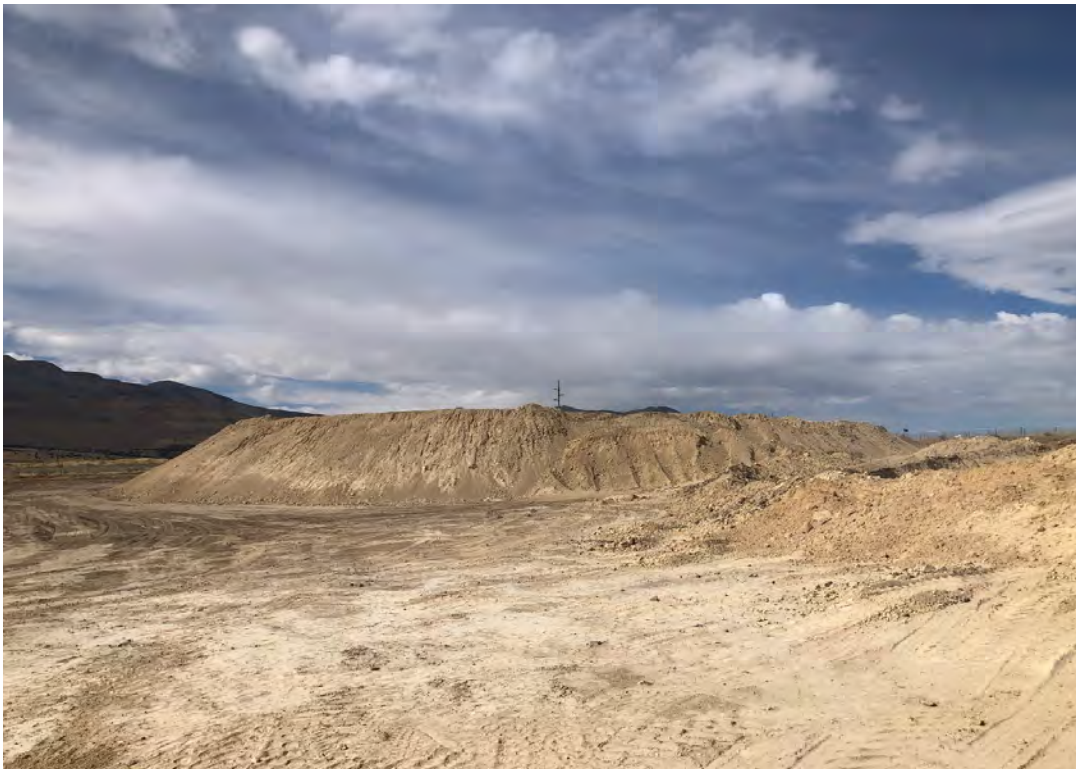
Stockpiled soil to preload the west tank
