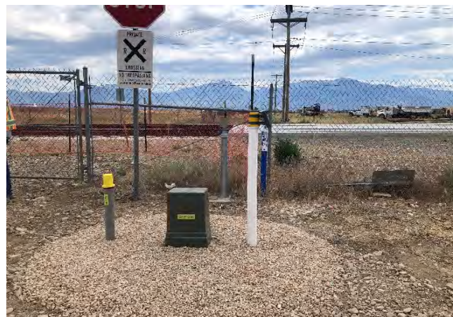
MetriCorr monitoring equipment and DC blocker
