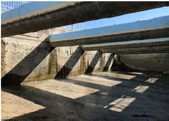
Basin effluent pipes to be replaced as part of this project
