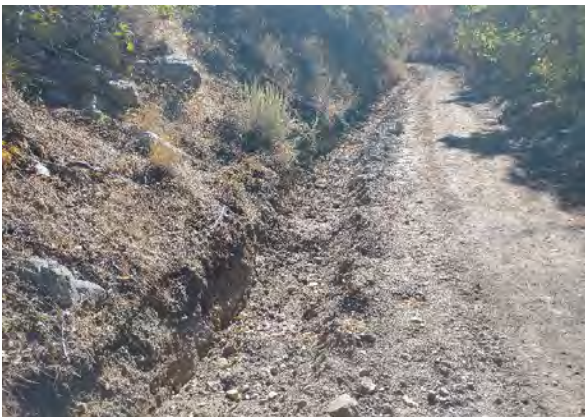
One of road storm drainage channels dug for project
