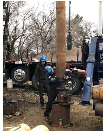
Installing column pipe for test pump
