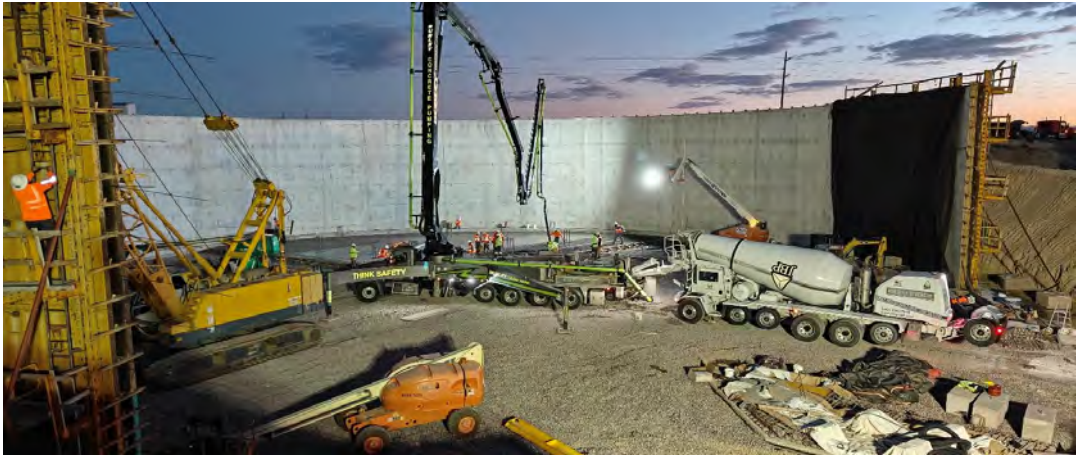
Early morning concrete placement
