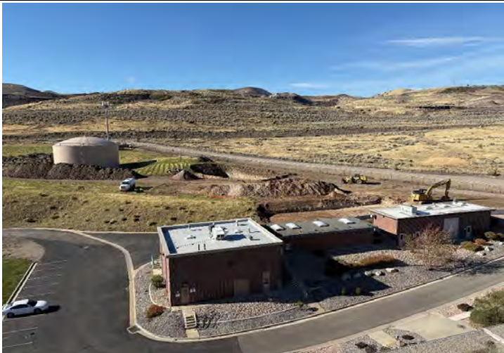
Foundation excavation for disinfection building and pH adjustment building
