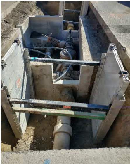
Old vault exposed and prepared for demolition work
