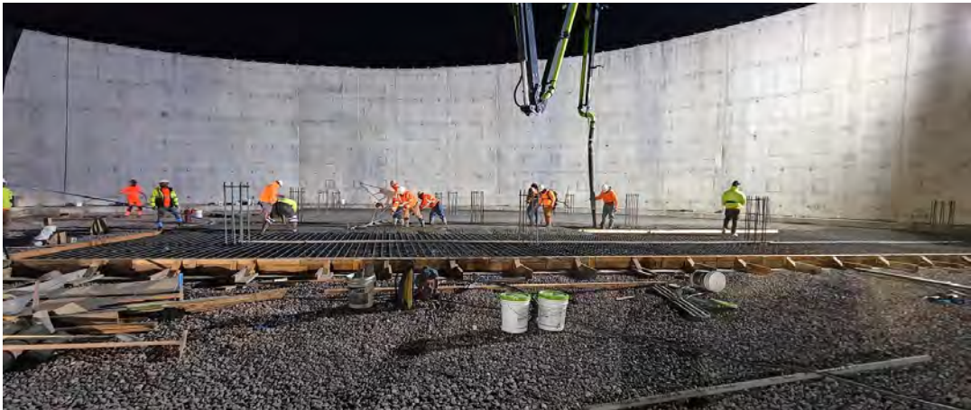
West tank floor slab placement
