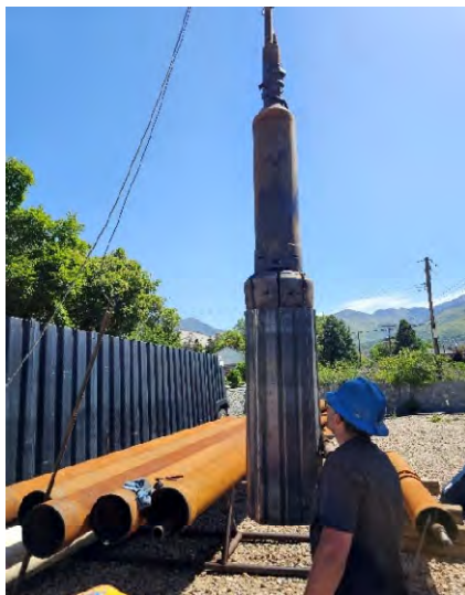
Installing well swage
