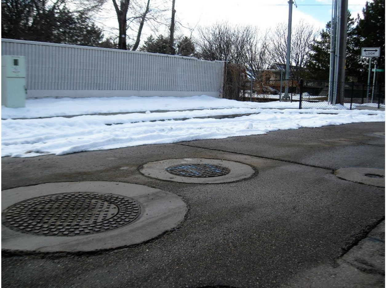
7500 S 175 W Vault
