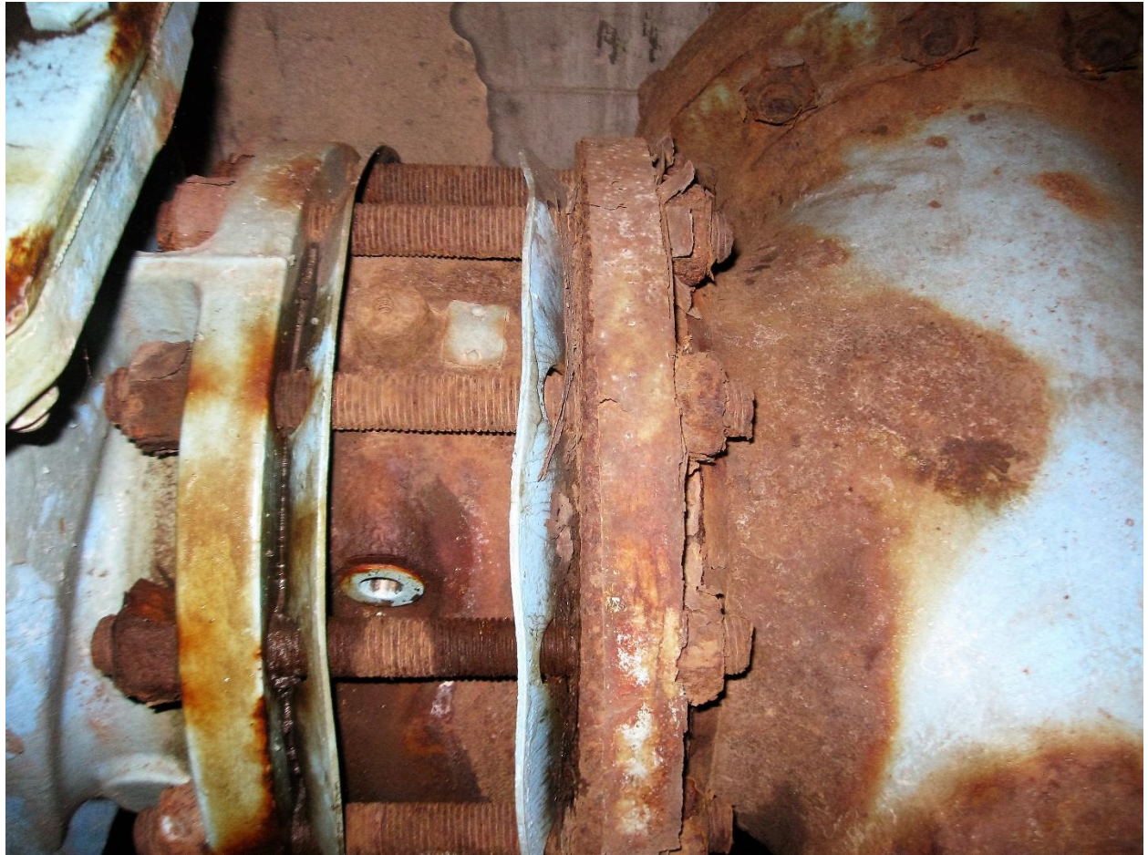
7500 S 175 W Vault
