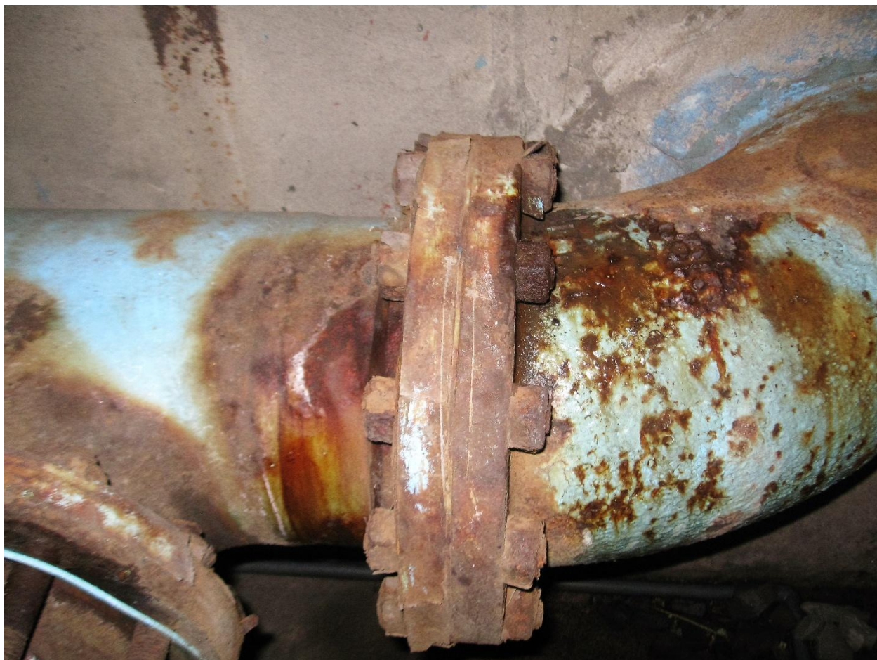
7500 S 175 W Vault
