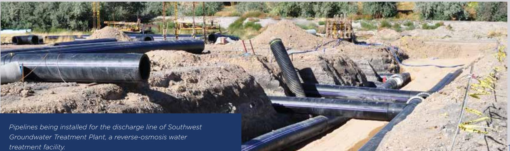
*Pipelines being installed for the discharge line of Southwest Groundwater Treatment Plant, a reverse-osmosis water treatment facility.*
