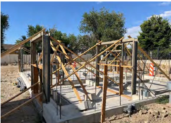
Door frames set, ready for block walls at 700 East
