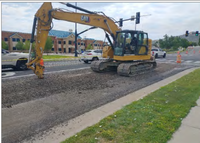
Preparing road for pipeline installation
