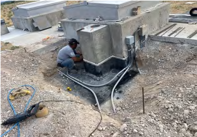
Liner installation
