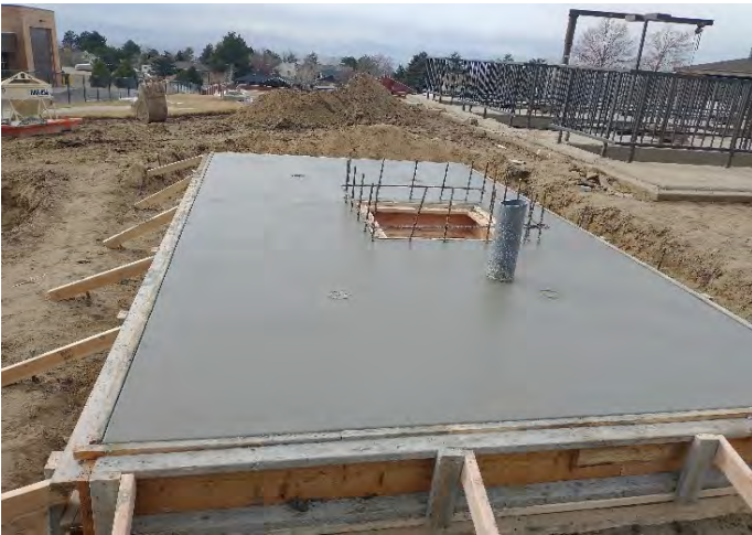
Newly poured vault influent vault roof
