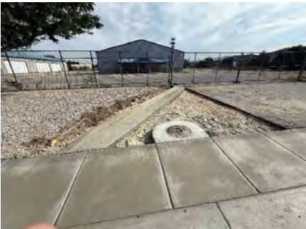
ISF concrete work east entrance
