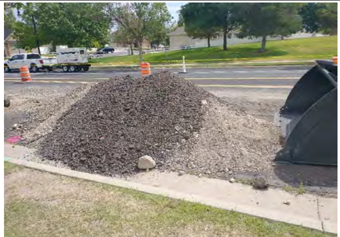
Stockpiled material on-site for pipeline installation
