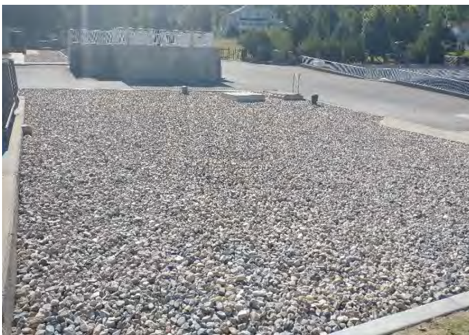
New landscape rock above completed influent vault to replace turf grass
