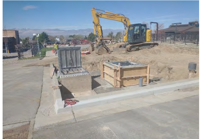
Influent vault with new roof and hatch
