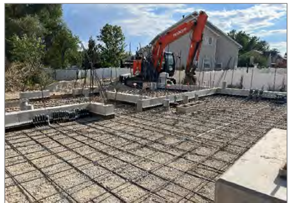
Rebar mat at 1000 East
