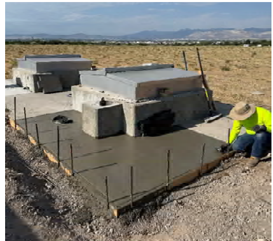
Concrete sidewalk installed
