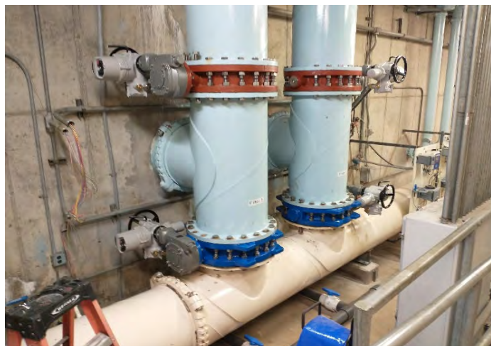
New Valves and actuators in filter gallery
