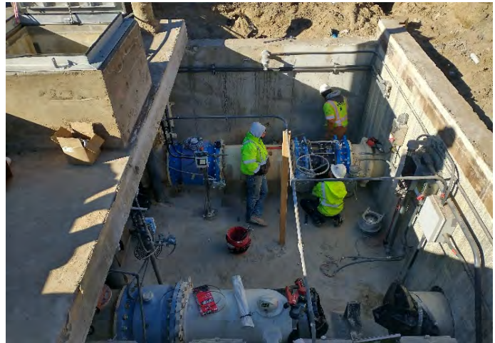
Removing valves in influent vault
