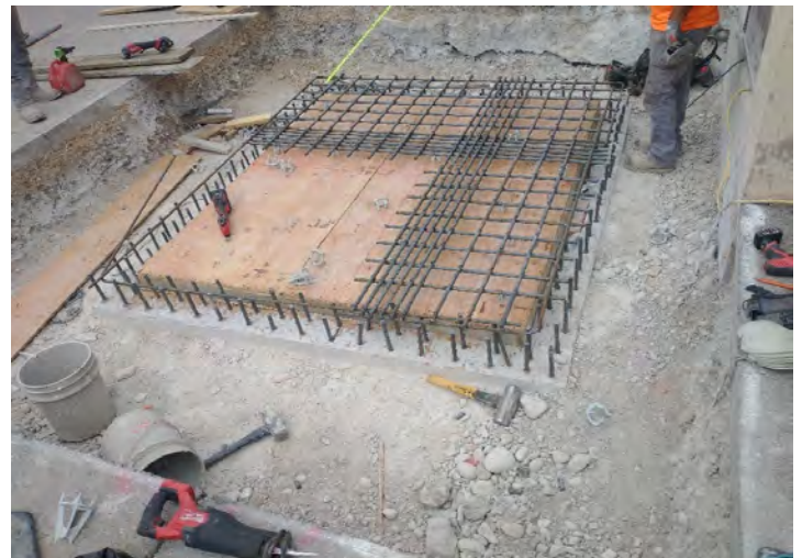
Forming rebar for new roof to vault at 6200 South 3200 West site
