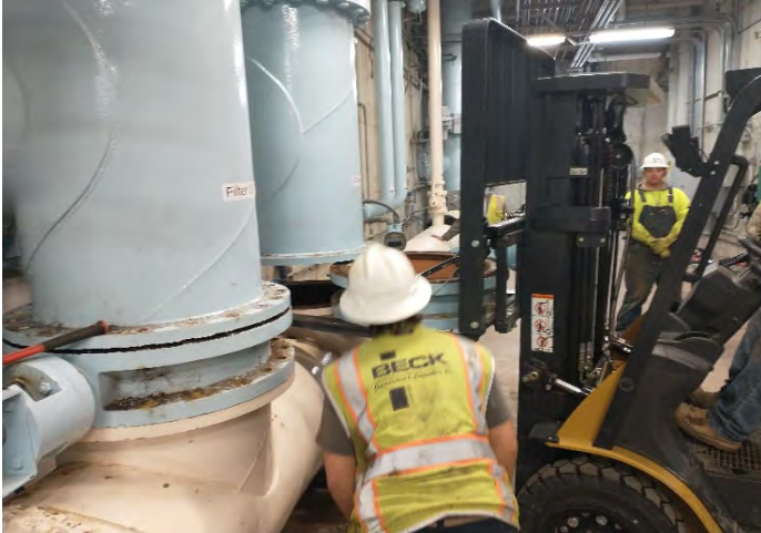
Removing old valves in filter gallery
