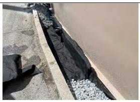
Placement of gravel around the base of the 8-MG reservoir
