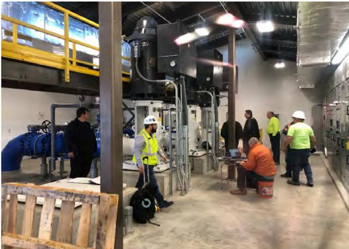
Electrical bump test of the new pump motors
