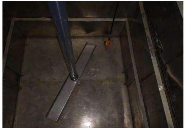
Inside the new batch tank with mixer and float
