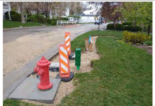
Completed new service meter box, new sample station, and new hydrant
