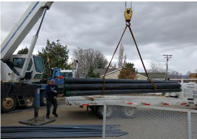
Installing new column pipe in well
