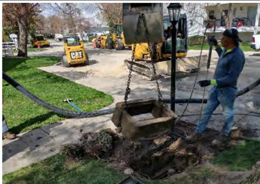
Replacing meter boxes at service connection
