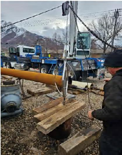
Setting up instrumentation to perform casing log
