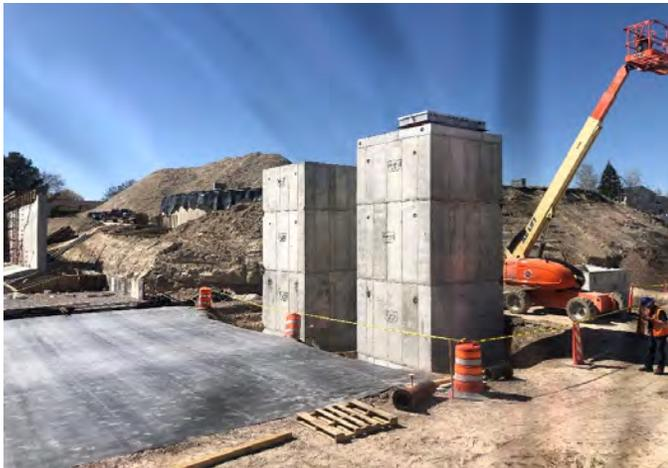
Construction of the reservoir overflow and drain box
