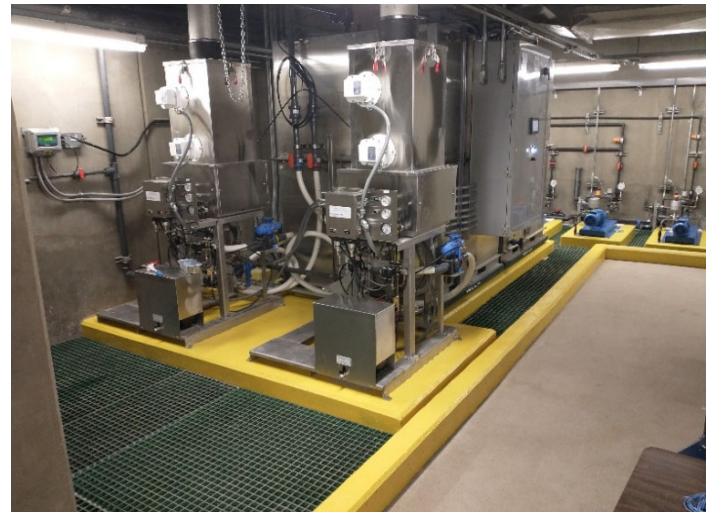
Completed New Polymer System
