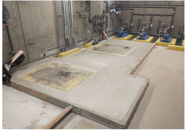
Forming Concrete Pads for New System
