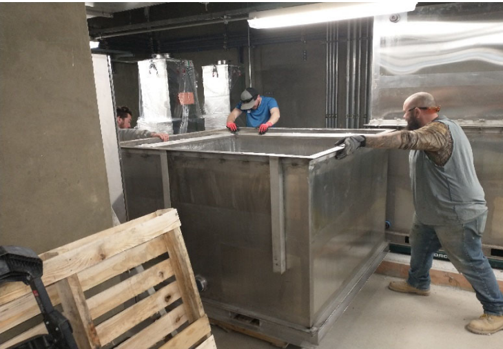
Installing New Bulk Tanks
