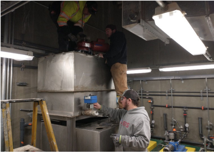
Original Polymer Bulk Tanks
