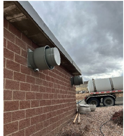
New exhaust fans on Alum Building
