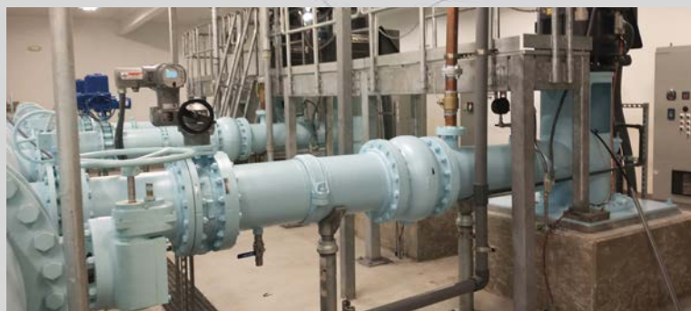
Refurbished Vault at 2200 W and 6200 S
