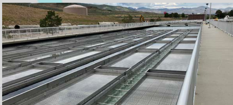
JWTP Sedimentation Basins Equip. Replacement
