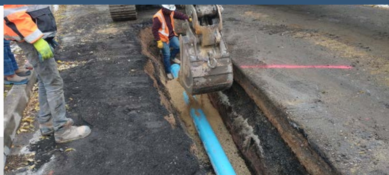
Distribution Pipeline Replacements - Redmaple Area
