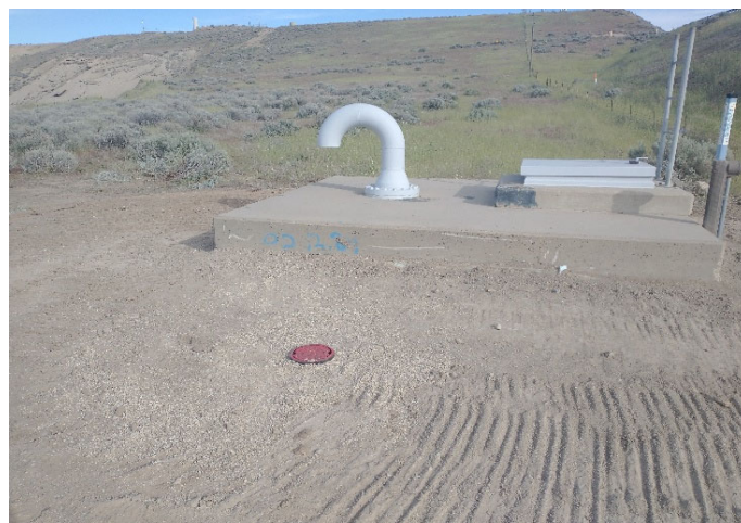
Restored vault area
