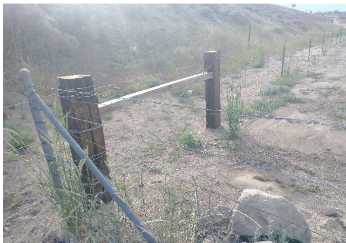
Restored field fence
