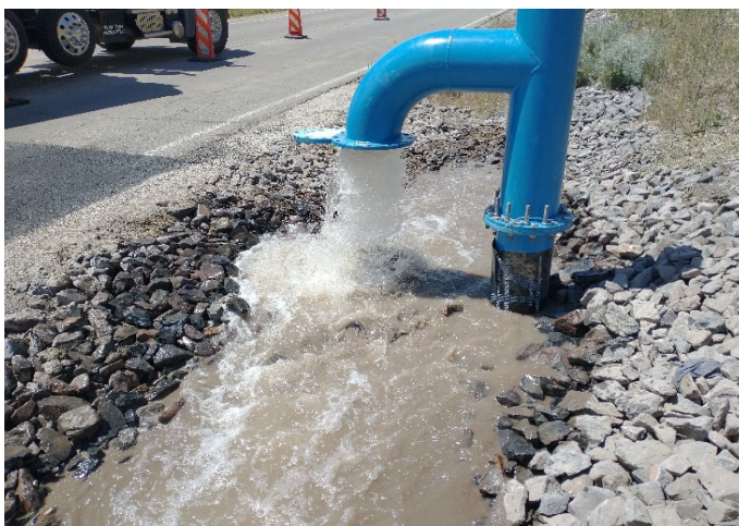
Testing of new blowoff
