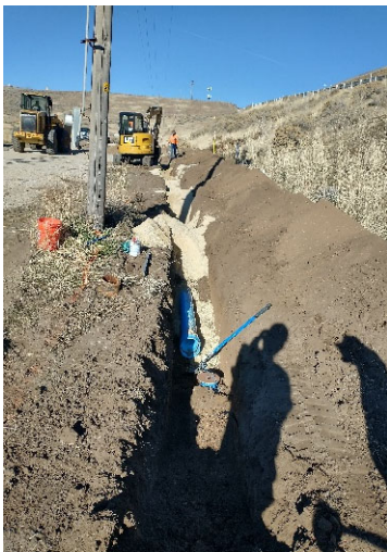
Installing new pipe in trench
