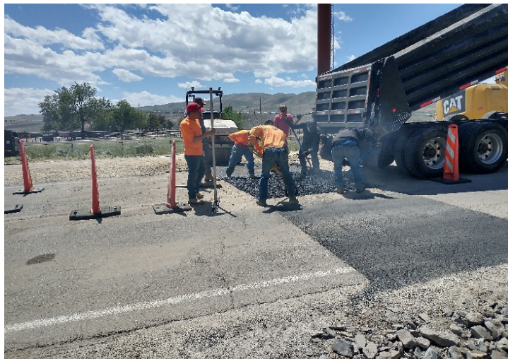
Asphalting road crossing
