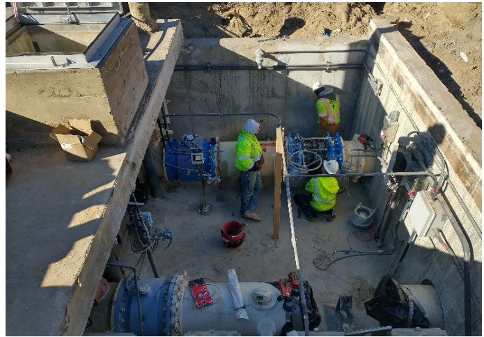
Removing valves in influent vault
