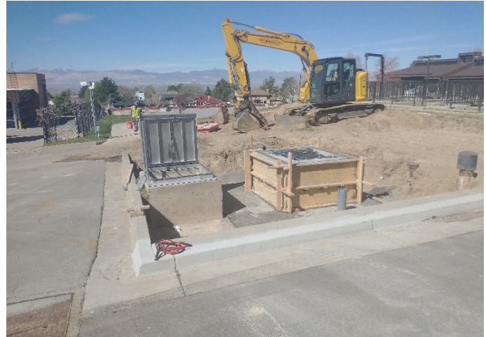
Influencer vault with new roof and hatch
