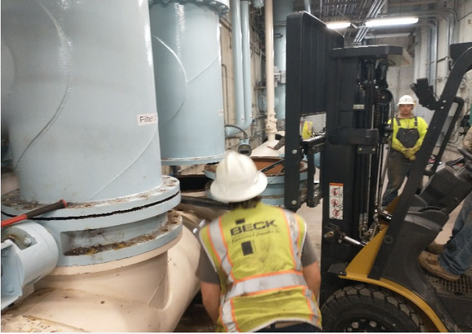
Removing old valves in filter gallery
