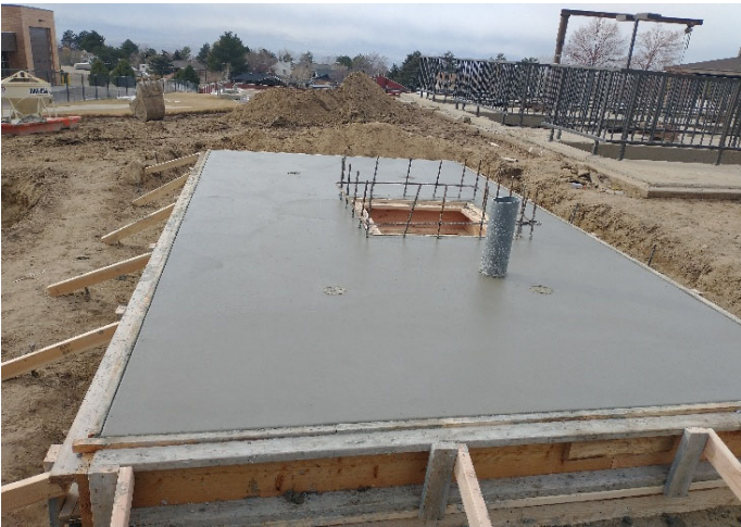
Newly poured vault influent vault roof
