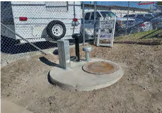
New air-vac vault constructed on 300 West 4320 South
