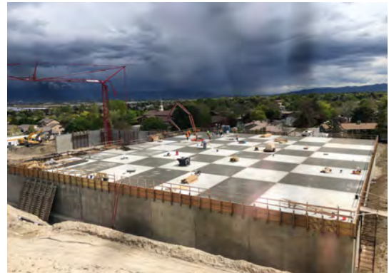
Concrete roof panels being poured
