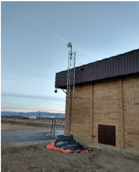
Tower constructed to move communication equipment off roof prior to booster pump station construction
