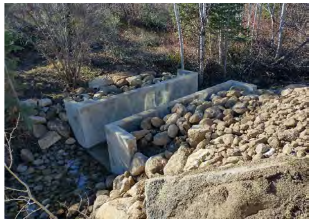
The fully formed flume in place
