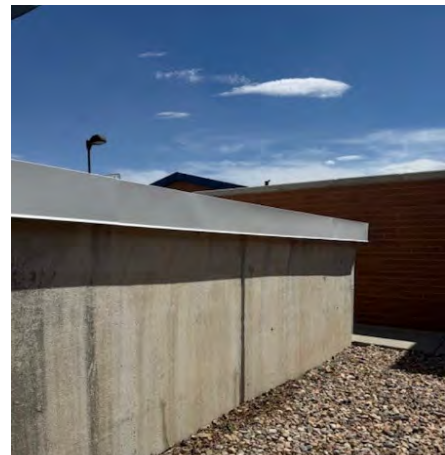
New perimeter flashing
