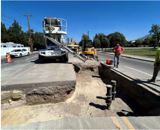
New 12" and 8" gate valves in 1300 E
