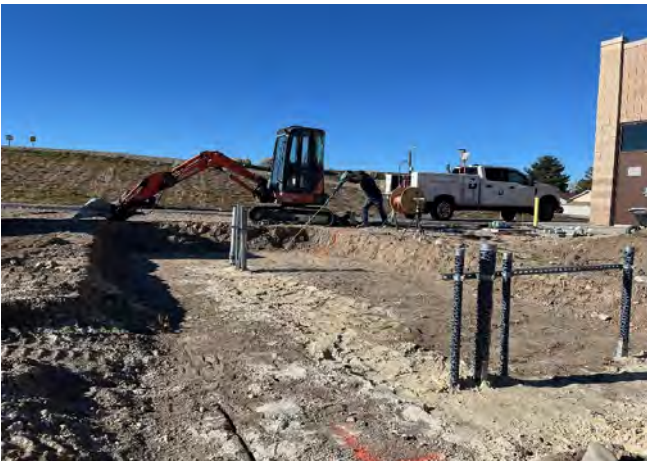
Conduits for the generator pad at the Terminal Reservoir site
