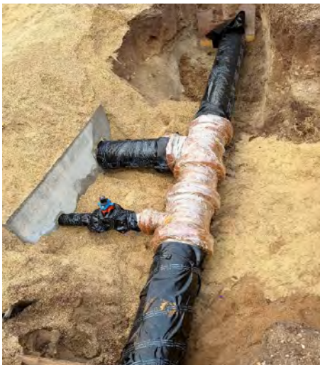
New 14-inch well discharge piping
