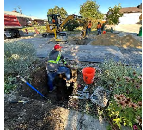
Installation of new meter box on 1430 E
