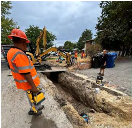
Installation of new hydrant on Hemmingway Drive
