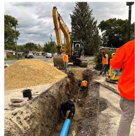
Connecting into existing line on Hyland Lake Drive
