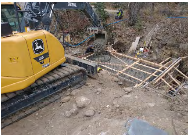
Placing concrete for flume base in streambed
