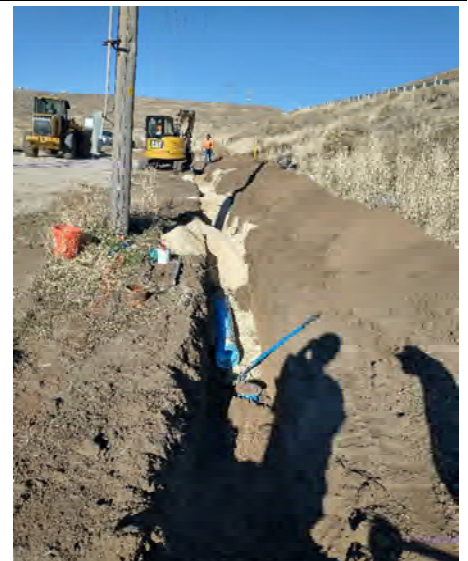
New drain line being installed in trench
