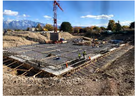
Setting forms and rebar for reservoir floor
