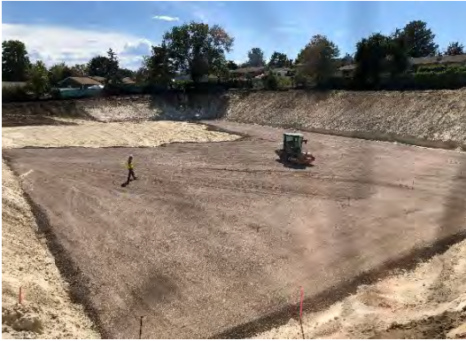
Preparation of reservoir subgrade
