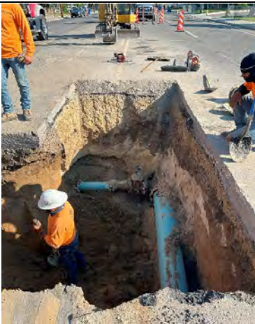
Worker uncovering existing pipe for tie in along 1300 East
