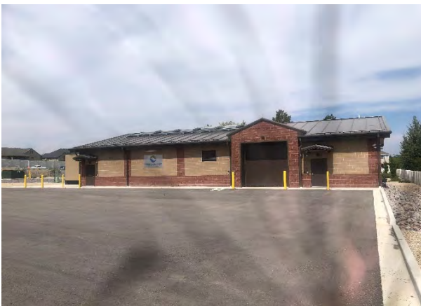
Finished gallery level
