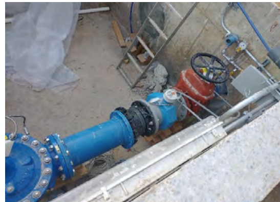
New meter and valves in vault
