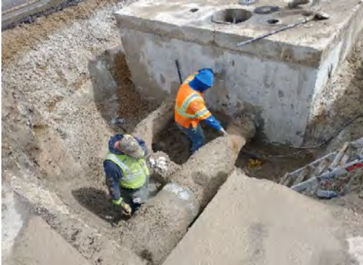
Excavating the vault and piping
