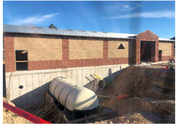
Installation of the surge tank and construction of the main level
