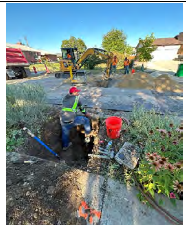
Worker reconnecting service lateral along 1430 East
