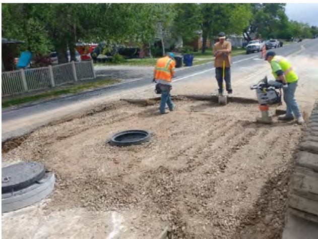
Backfilling and compacting over vault
