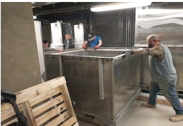
Installing new bulk tanks
