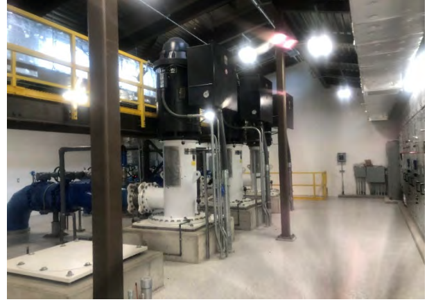
Finished gallery level
