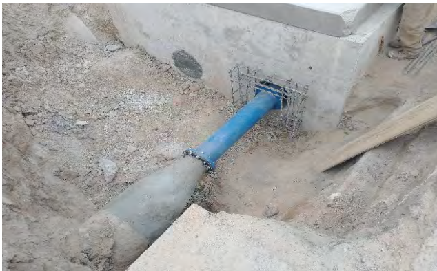
New piping attached to pipeline with thrust block being formed
