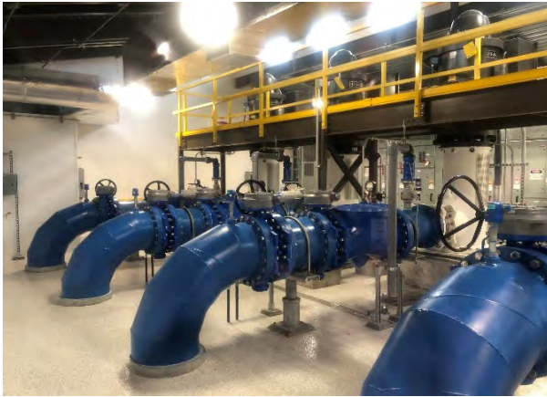
Construction of the well house piping in the gallery level
