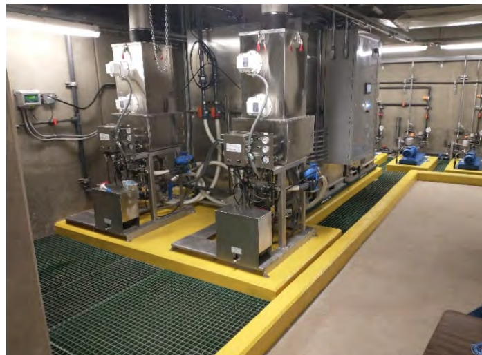
Completed new polymer system
