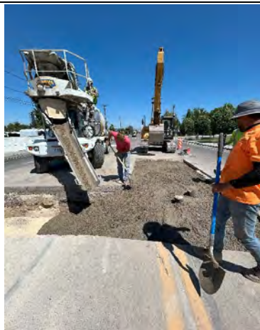
Contractor pouring flow fill on 1300 East after completed tie in
