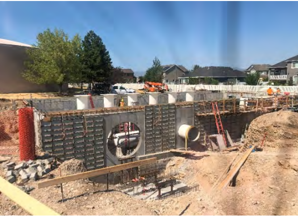
Construction of the well house piping in the gallery level
