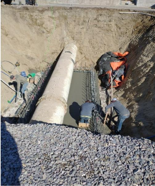
Excavated effluent pipeline with new vault floor poured
