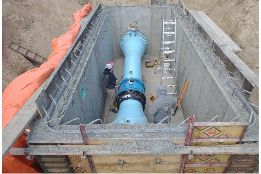
New effluent meter and piping installed in new vault
