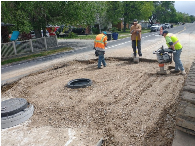
Backfilling and compacting over vault
