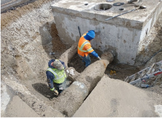
Excavating the vault and piping
