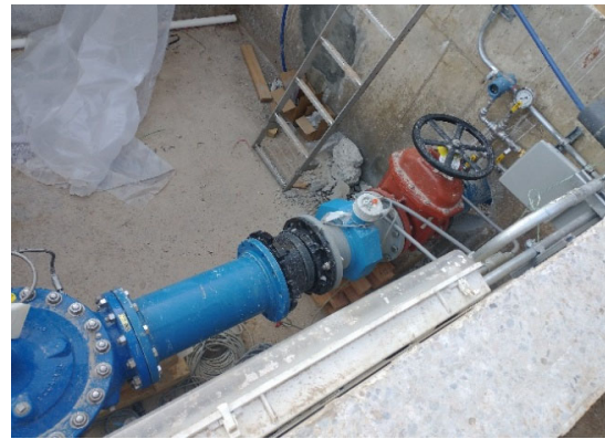
New meter and valves in vault
