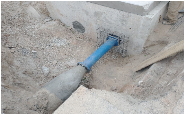
New piping attached to pipeline with thrust block being formed
