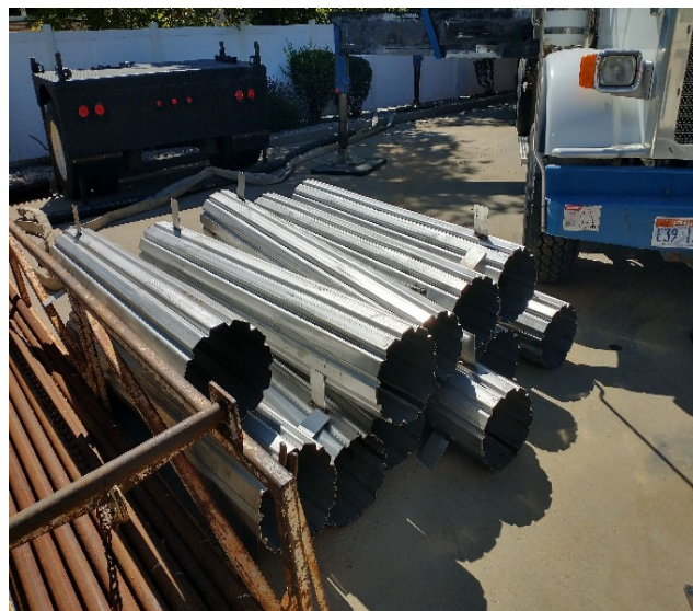
Well casing patches before installation
