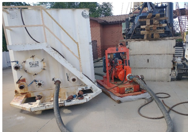
Chemical treatment equipment
