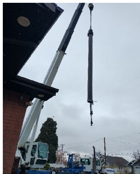
Re-installing the pump column
