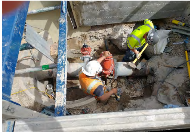
Installing new valves and welds
