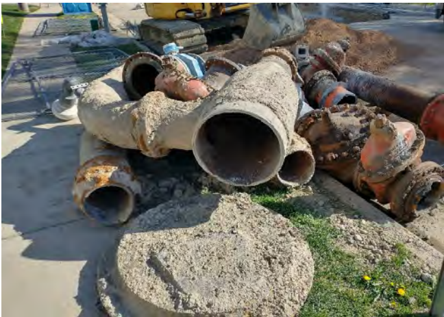
Old pipe and material removed from the vault
