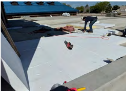
Geofoam placed on to of the CCB
