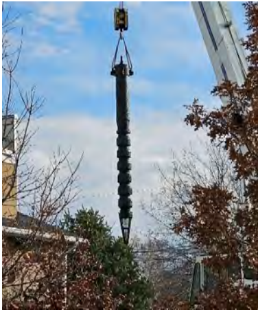
Pulling the existing pump
