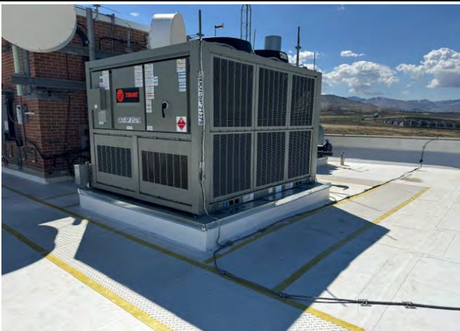
New Chiller installed at the JWVTP high-rise
