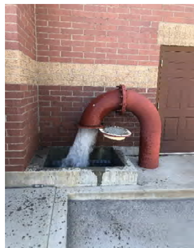
Pumping to waste during start-up
