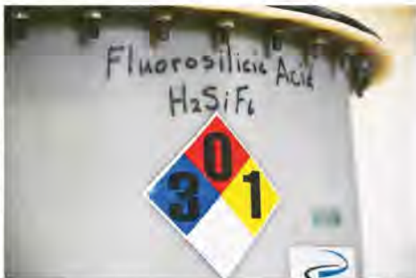
The smaller day storage tank of fluorosilicic acid at one of Weber Basin Water Conservancy District's nine locations in Layton is pictured on Monday.
