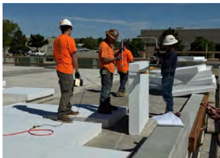
Workers cutting the geofoam to size
