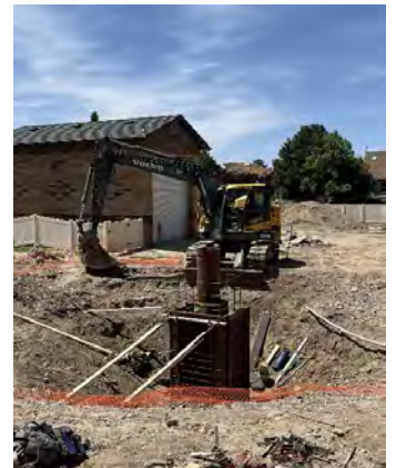
Installing new pipe and valves in the vault
