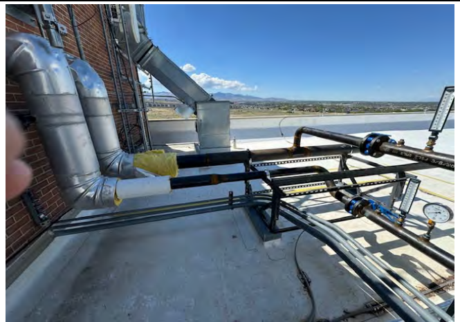
New piping for the newly installed chiller
