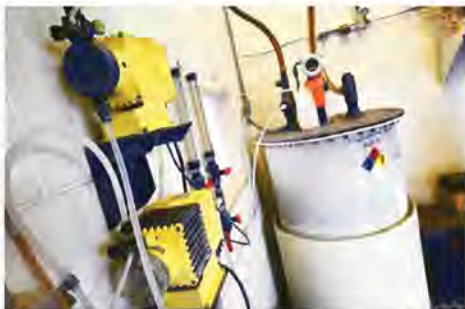
Dosing pumps inject fluoride into carrier water at one of nine Weber Basin Water Conservancy District locations in Layton on Monday.
