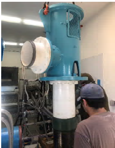
Installing the pump discharge head
