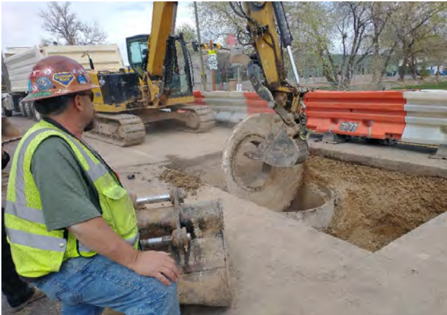
Demolishing old vault in roadway
