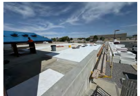
Geofoam adhered to CCB deck
