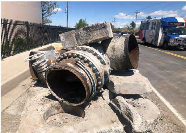
Demolition of the existing piping and vault lid
