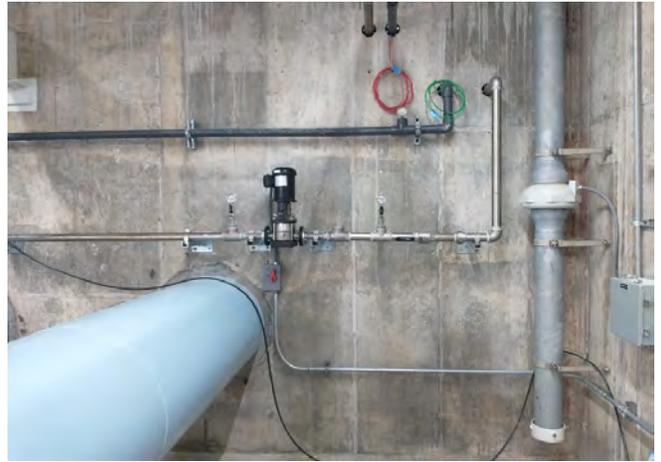
Circulation pump in vault operating new chemical feed line
