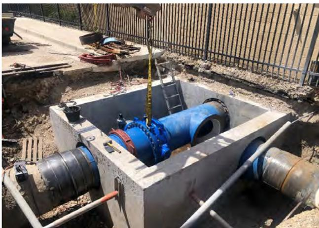
Installation of the new 30-inch piping and valves
