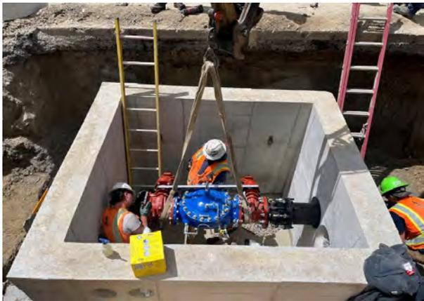
Installation of the new vault and pressure regulating valve at Gordon Lane
