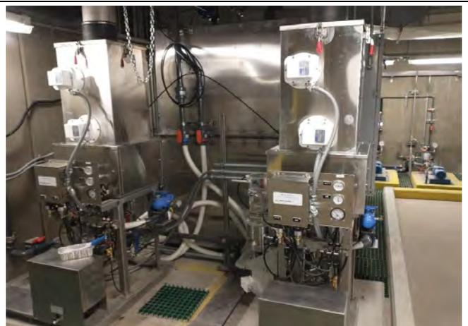
The fully installed dry polymer mixers and batch tanks
