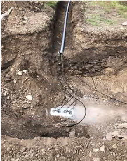
Cables cad welded to the 42-inch pipeline
