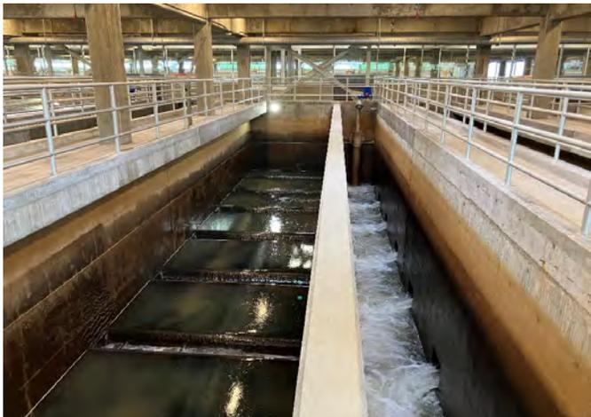
JWTP Filter to be upgraded with deeper media and increased flow rate as part of this project
