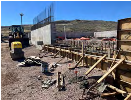
Last foundation wall for Chlorine Building being prepared
