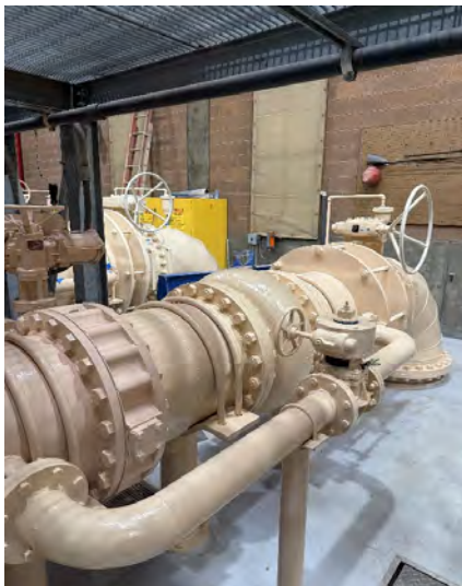
New valves and equipment installed and painted
