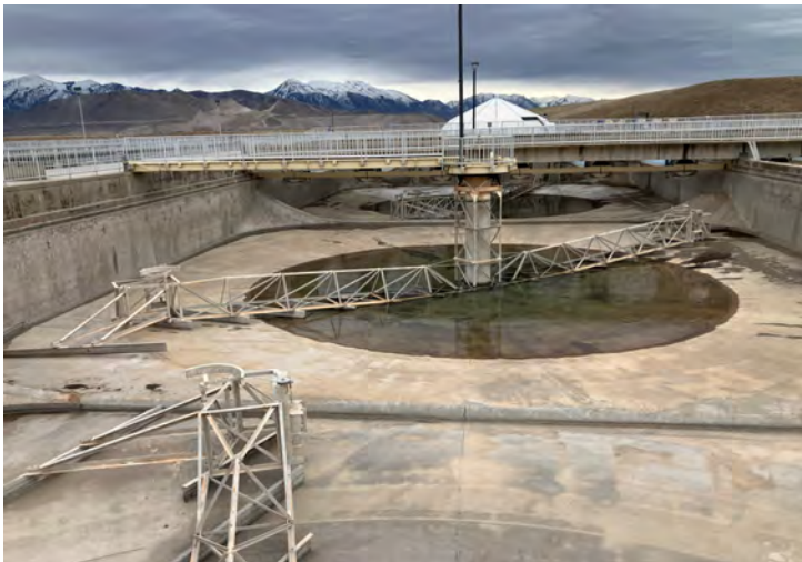
JWTP Basin 1 drained for inspection
