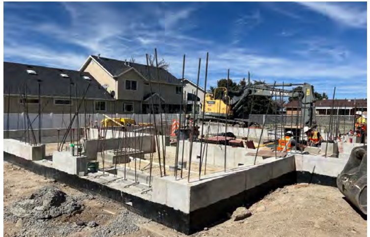
Foundation walls at the 1000 East site
