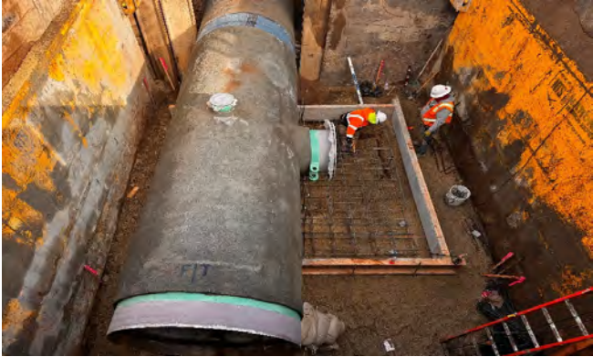
Tying rebar for air-vac vault
