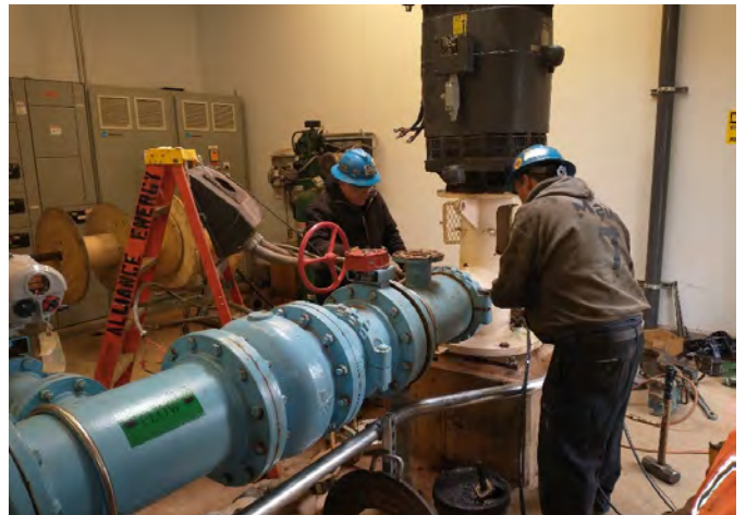
Installation of pump and motor
