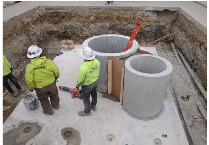
New vault lid installed on 110 East vault
