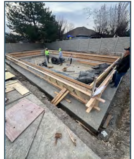
Setting forms for concrete foundation walls at 3145 West
