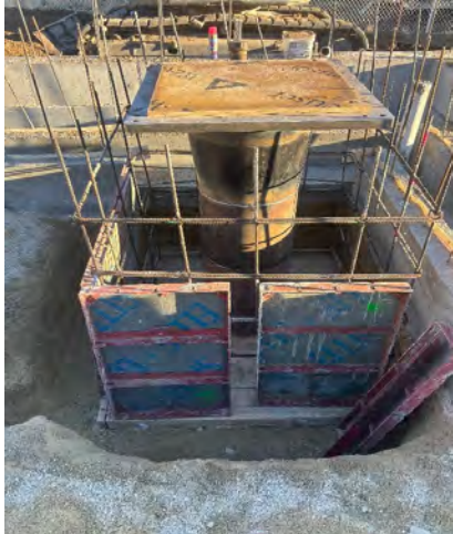
Welded sill plate to support pump equipment
