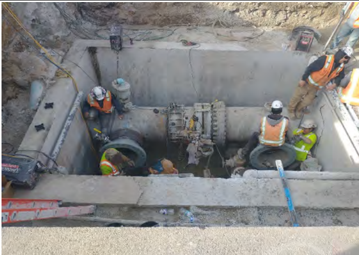
Replacing valves and piping in 110 East vault while lid is removed
