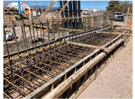
Reinforcing steel for Chlorine Building
