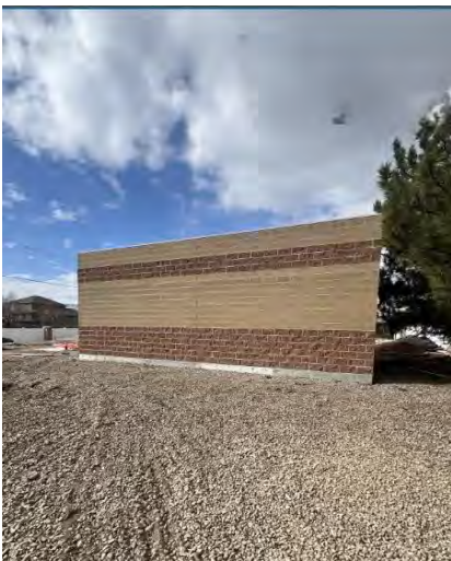
New generator sound/screening wall at 13400 South
