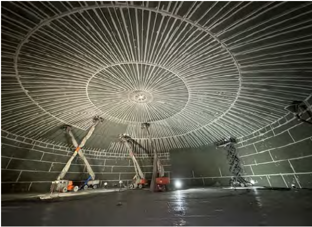
8-MG Reservoir interior painting
