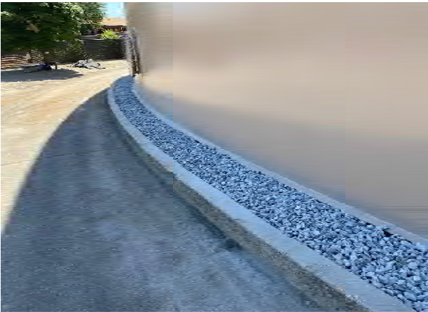
8MG Exterior New North Hatch
