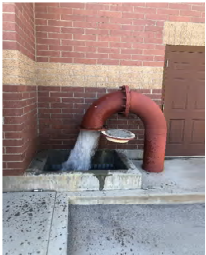
Pumping to waste during initial start-up
