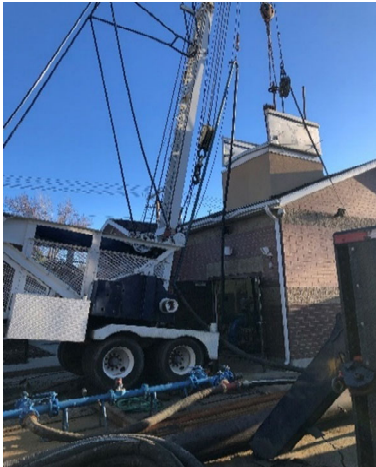
Well development rig
