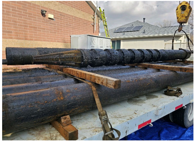
Existing pump and column pipe
