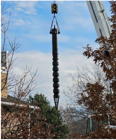
Pulling the existing pump
