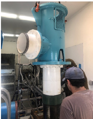
Installing the pump discharge head
