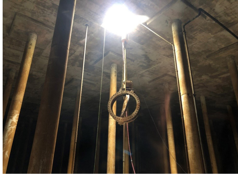
^ Terminal Reservoir Basin 2 Outlet Valve Replacement - removing the old 48" valve.
