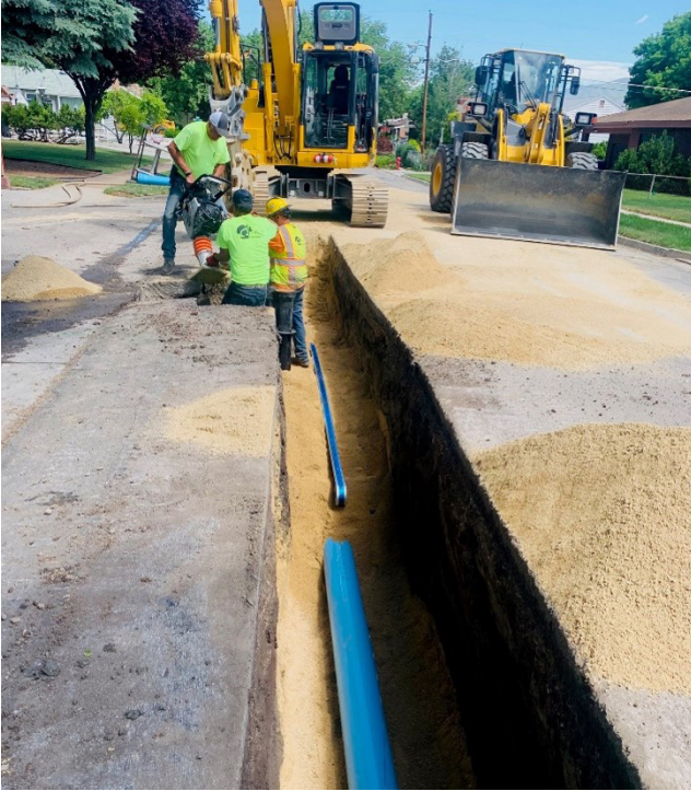
^ Millcreek & SSL Pipeline Replacements - Installation of the 8" pipeline along 610 East
