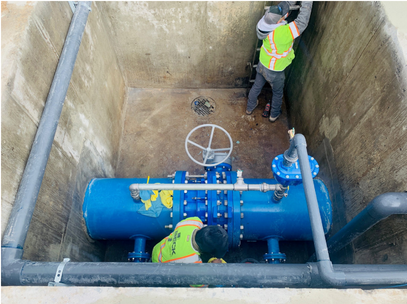
< 3600 W 4400 S Vault Project - New piping and valves
