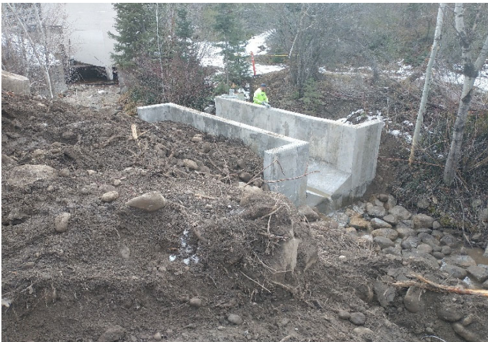
New concrete flume
