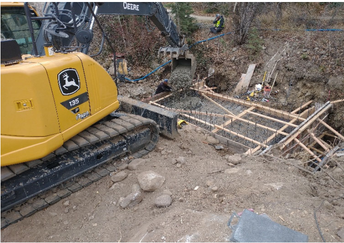
Placing concrete for flume floor
