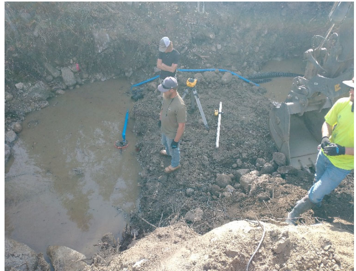
Forming base on flume in riverbed
