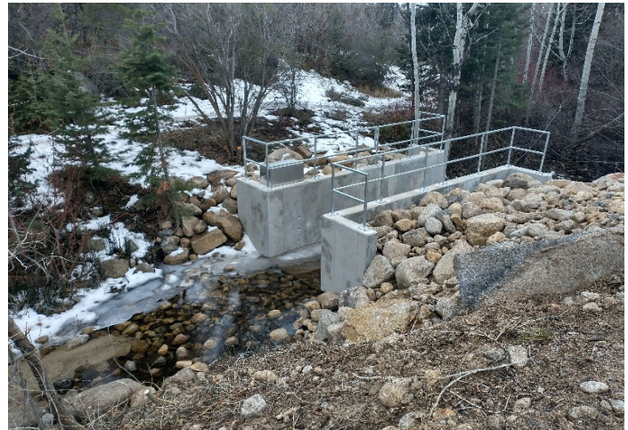
Completed flume with railings
