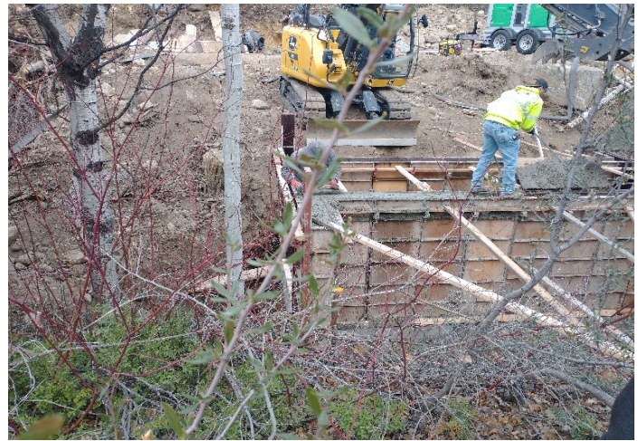
Placing concrete for flume walls
