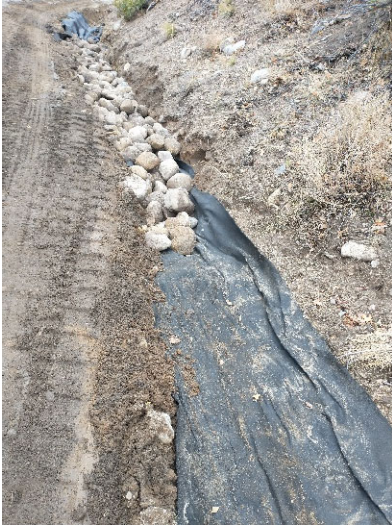
Laying riprap in new drainage channel
