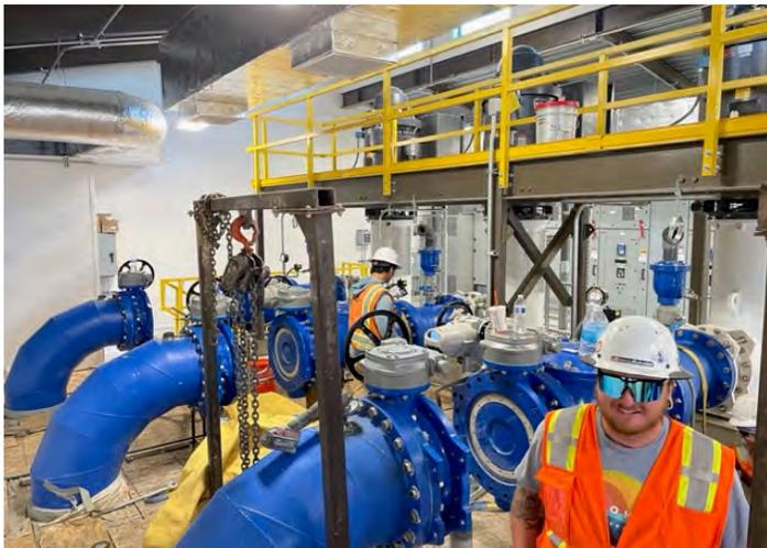
Modification of the discharge piping to eliminate air binding
