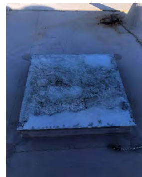
New galvanized steel skylight guards on the roof of the Chlorine Dioxide Building
