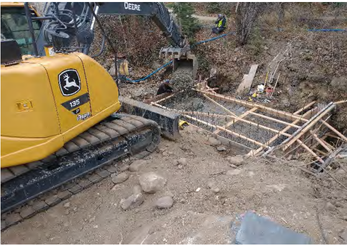
Placing concrete for flume floor
