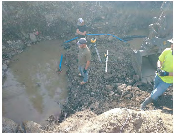
Forming base on flume in riverbed
