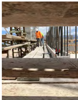
First course of concrete block for new Caustic Building
