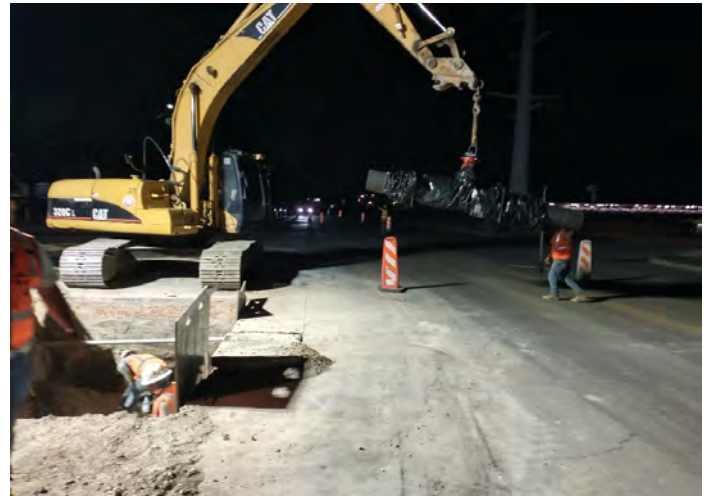
Installing new valve during nighttime shutdown on 900 East
