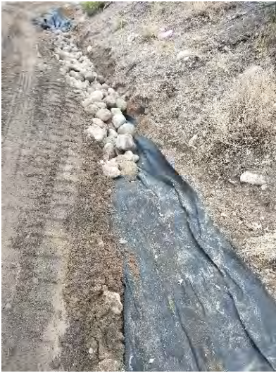
Laying riprap in new drainage channel
