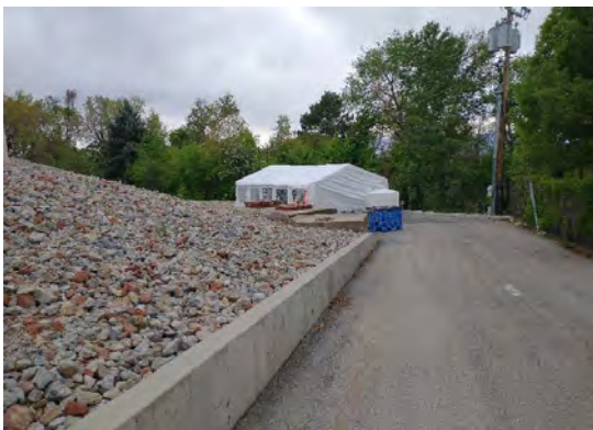
Pilot plant on reservoir site
