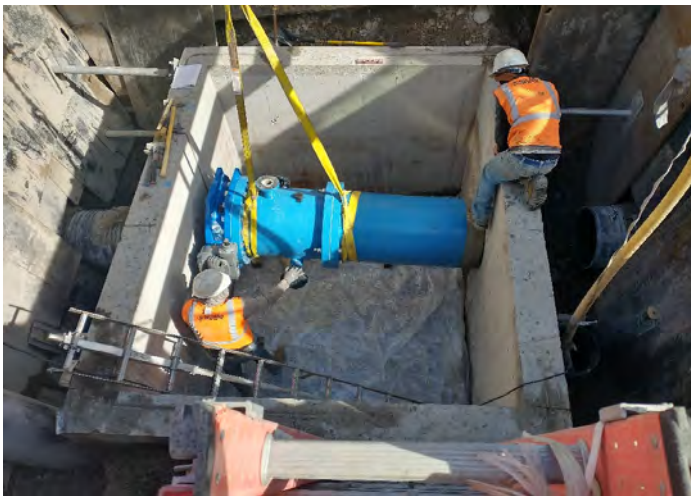
Installing new valve and piping at 4500 South vault
