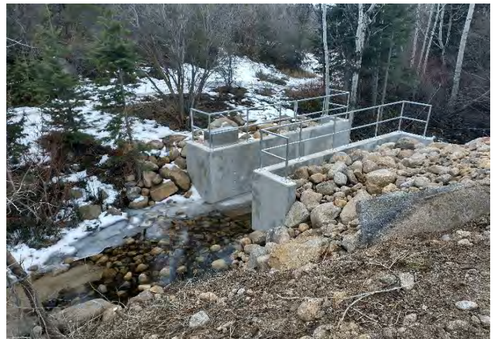
Completed flume with railings
