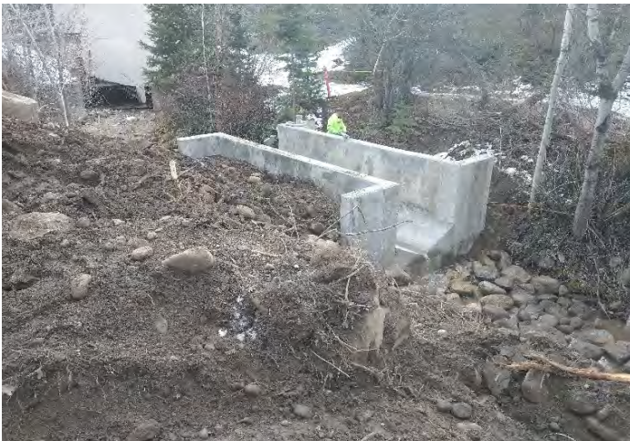
New concrete flume
