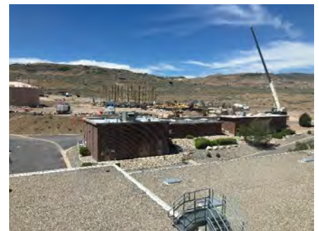
Safety scaffolding in place for masonry work on new Caustic Building
