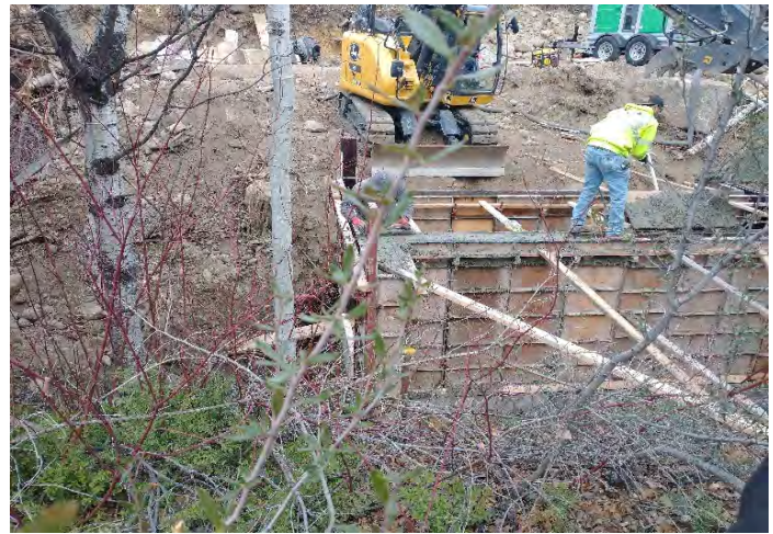
Placing concrete for flume walls
