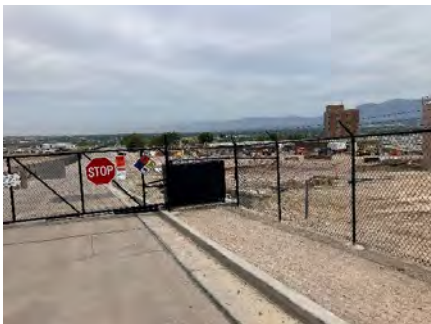
Newly relocated JWVTP south gate to secure site around the new buildings
