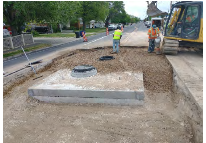
Backfilling the vault preparing for asphalt
