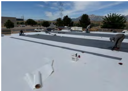
TPO and Protective Overlay Installation
