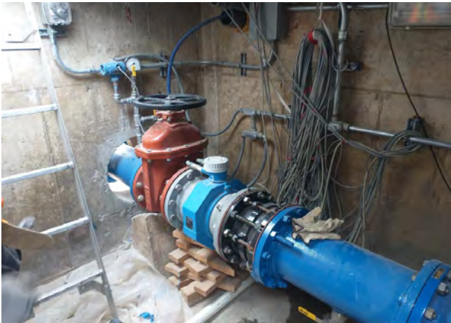
Newly installed flow meter with new valve and piping
