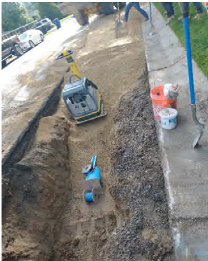
Workers backfilling trench along 5935 South
