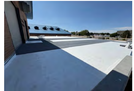
TPO Membrane and Protective Track Overlay (in dark grey)
