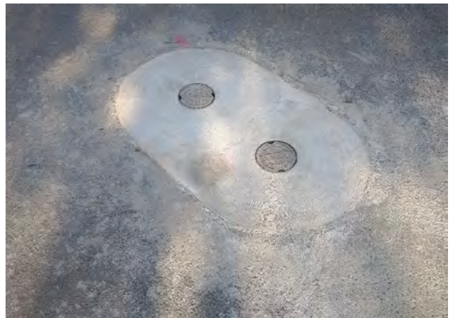
Former vault converted into buried valves
