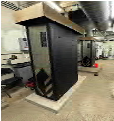
North View – Boilers over placed over concrete pads
