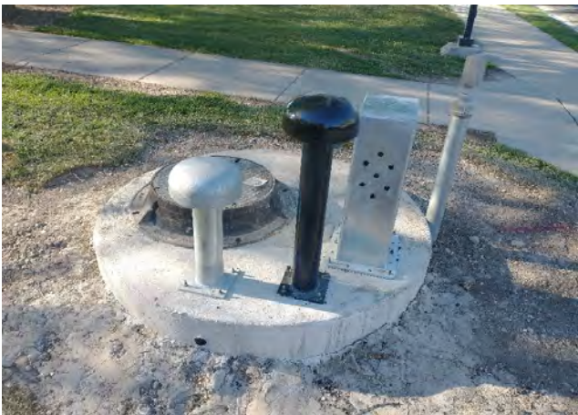
New air vac manhole constructed out of the street
