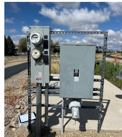
Upgraded electrical service
