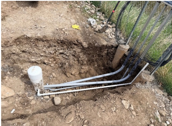
Electrical conduits being routed
