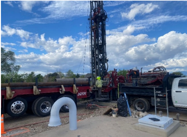
Drill rig to install anode wells
