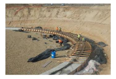
Setting forms and rebar for the East Tank footings
