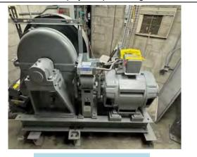
Elevator Motor and Gear
