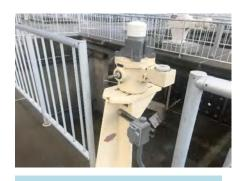
Flocculator motor to be replaced as part of this project
