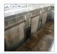
Setting forms and Aged influent gates to be replaced as part of this project for the East Tank footings
