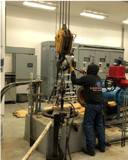
Adjusting hydraulic swage to patch the breach in the well
