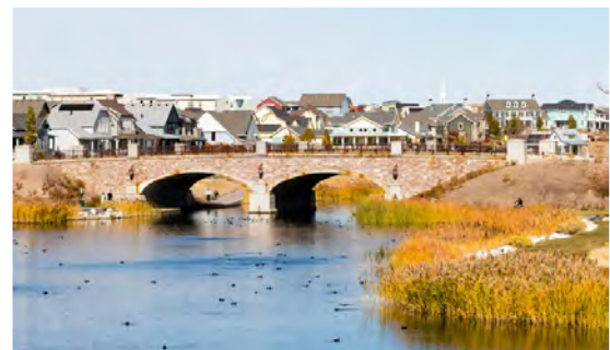
Response actions “bridge” the gap during water shortages
