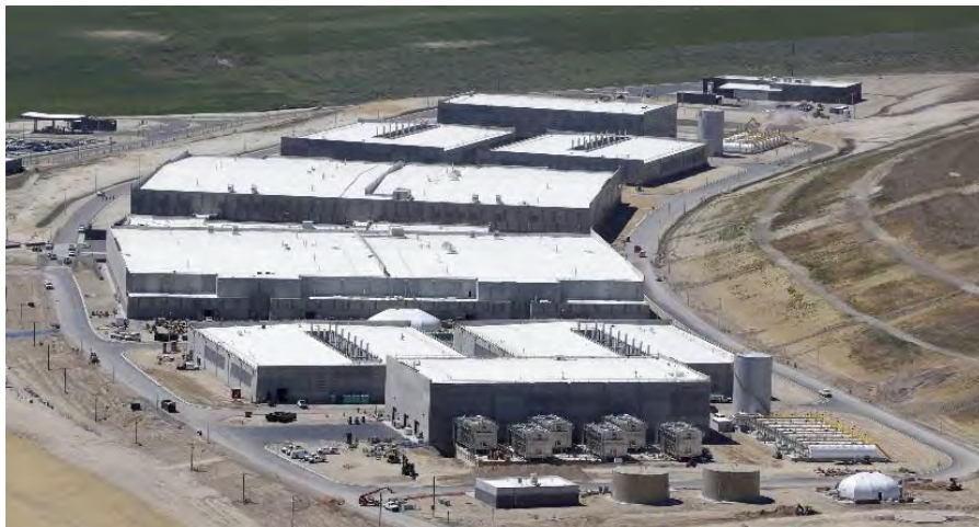
Figure 2-1. Data centers continue to grow in the region
