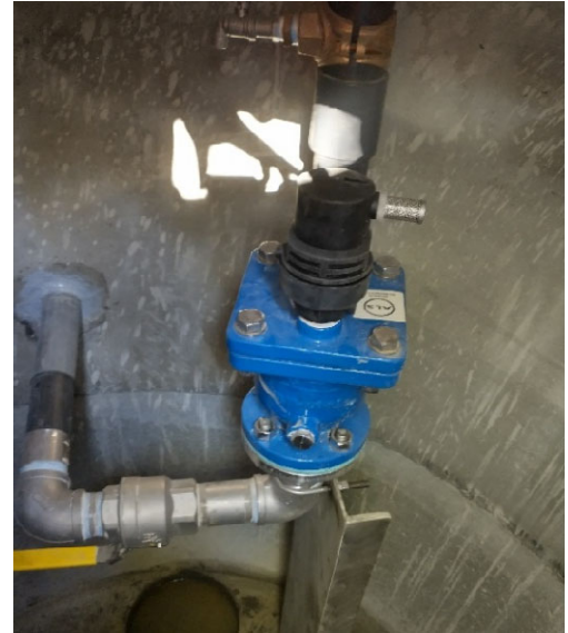
New air vac valve at 4390 S 2200 W
