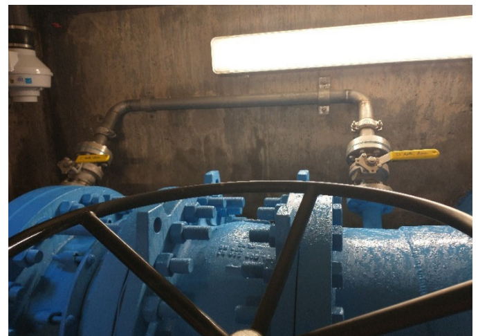
New mainline valve at 110 E 11400 S
