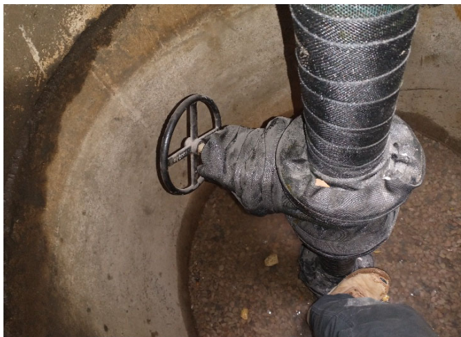
New valve and pipe at 4500 S 350 E
