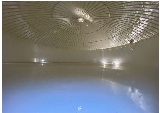
8-MG Reservoir interior painting
