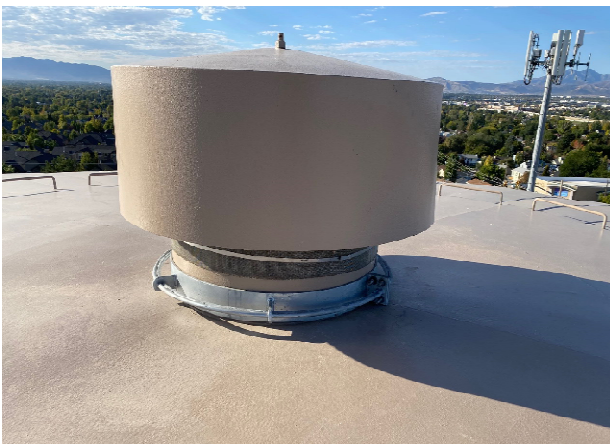
8MG New Vent and Fall Arrest System
