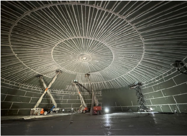
8-MG Reservoir interior painting
