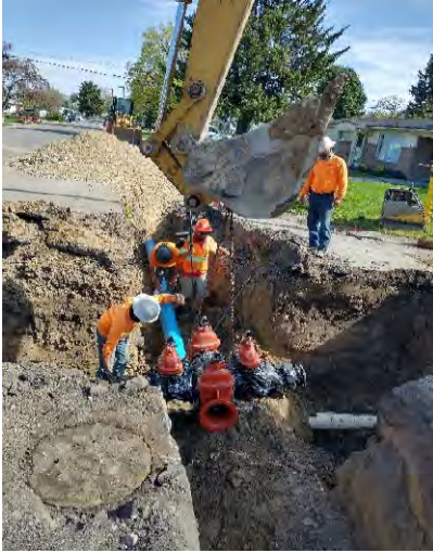
Installing new 4-valve cross in Murray
