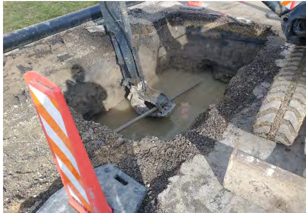
Drilling under creek in Old Farm
