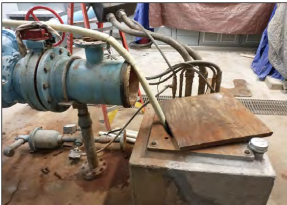
Running water down the well to prepare for the well video
