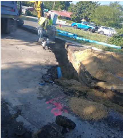
Laying new pipeline in roadway
