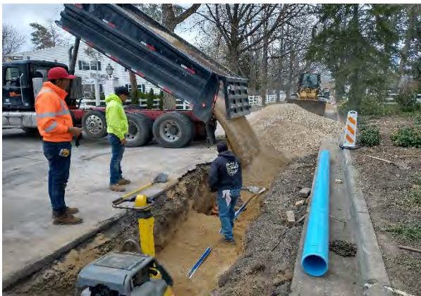
Backfilling pipeline in Old Farm
