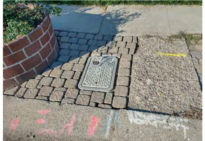
Replaced meter box with restored landscape
