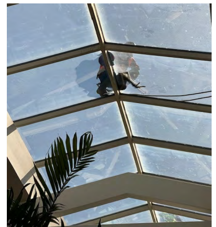
Worker Replacing the Skylight Sealant
