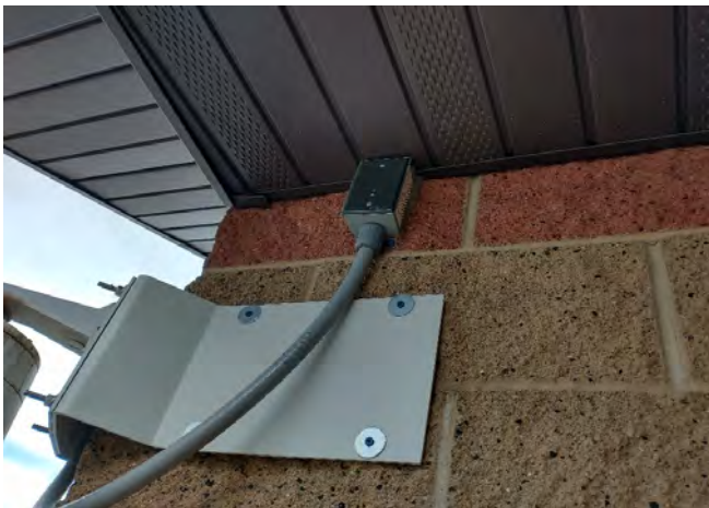
Electrical box on building outside sealed
