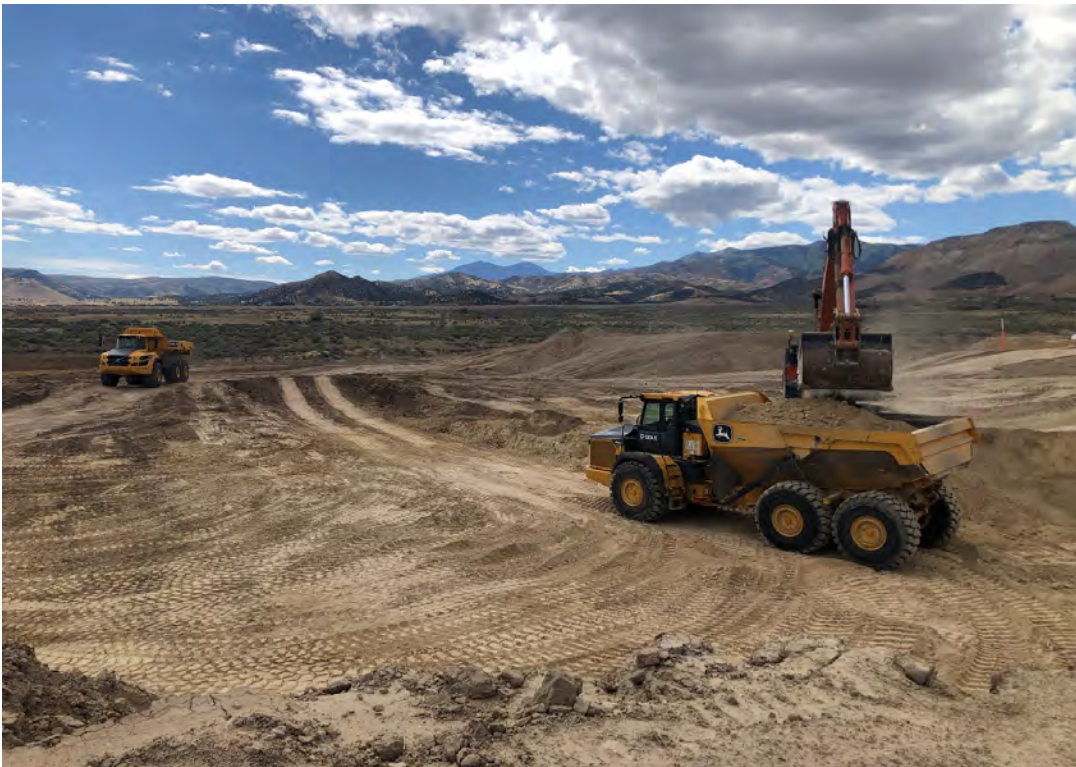
Removing overburden to excavate to the subgrade on the east tank
