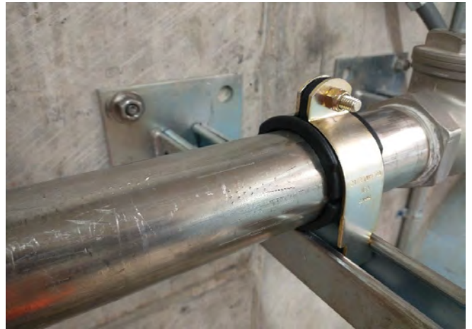
Pipeline clamp coating to prevent corrosion
