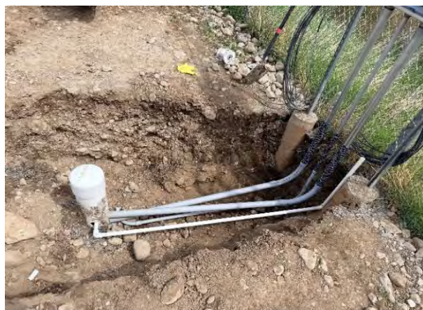
Electrical conduits being routed
