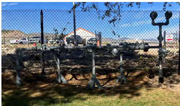
Enbridge has completed the natural gas service line replacement to JWTP
