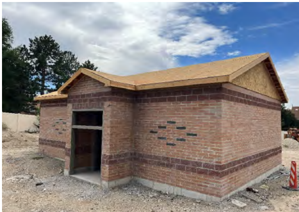
Roofing installed at the 700 East site
