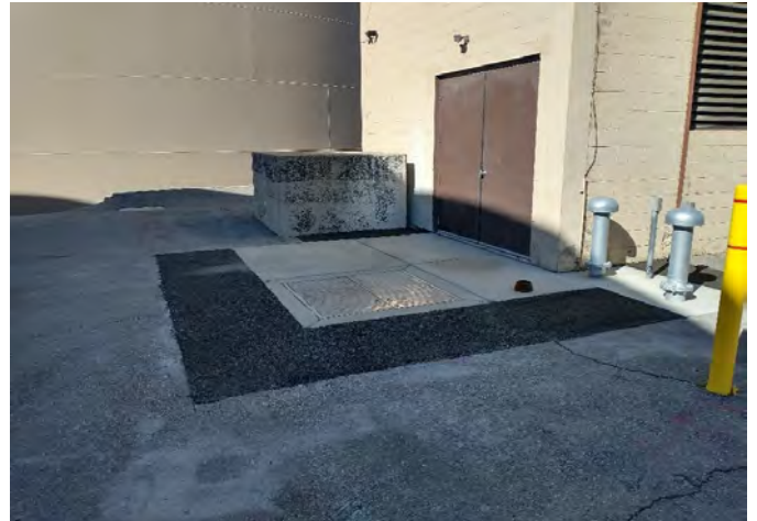
New concrete and asphalt over 6180 South 3200 West vault
