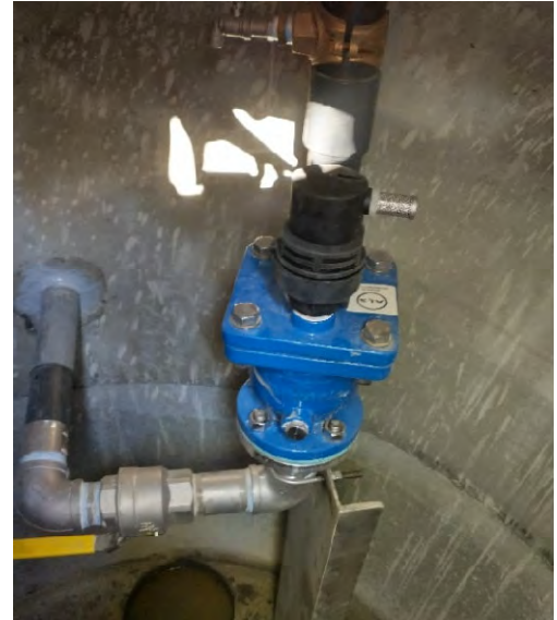
New air vac valve at 4390 S 2200 W
