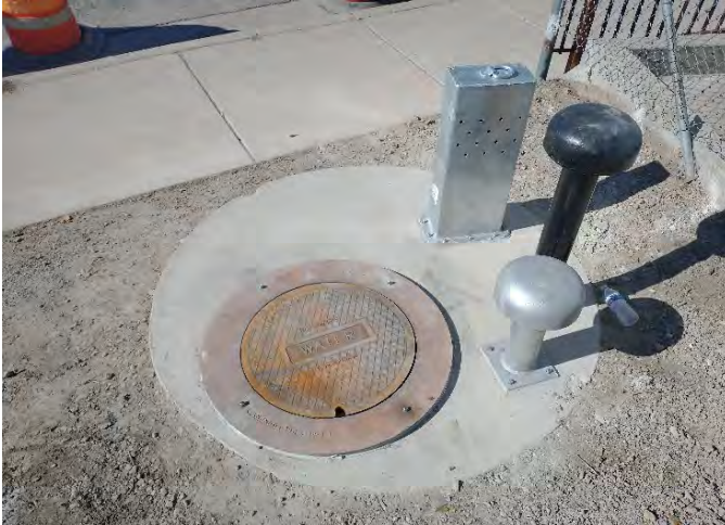
New manhole lid and vents at 4330 S 300 W
