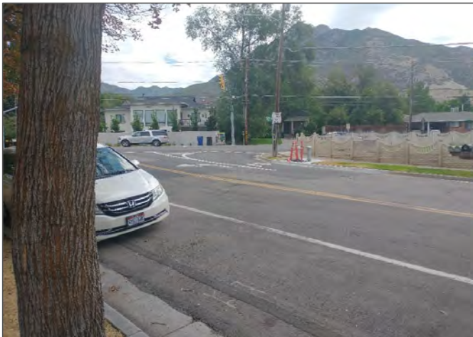
New asphalt, vent pad, and line stripping over Cottonwood's vault
