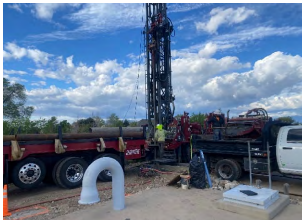
Drill rig to install anode wells
