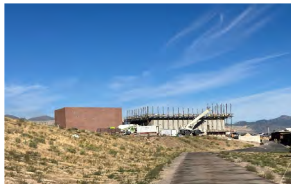
Caustic Building brick veneer has been placed. Masons are preparing to install brick veneer on the Chlorine Building
