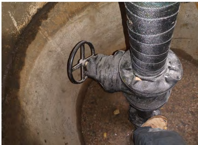
New valve and pipe at 4500 S 350 E
