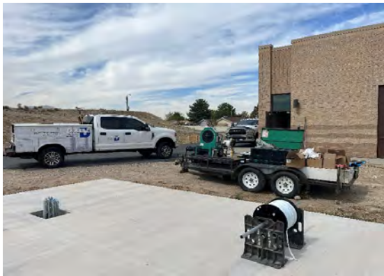
Preparing to pull wire for the generator installation
