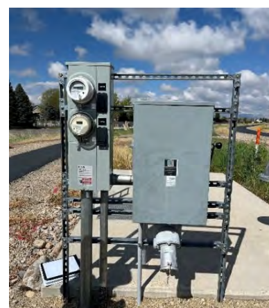
Upgraded electrical service
