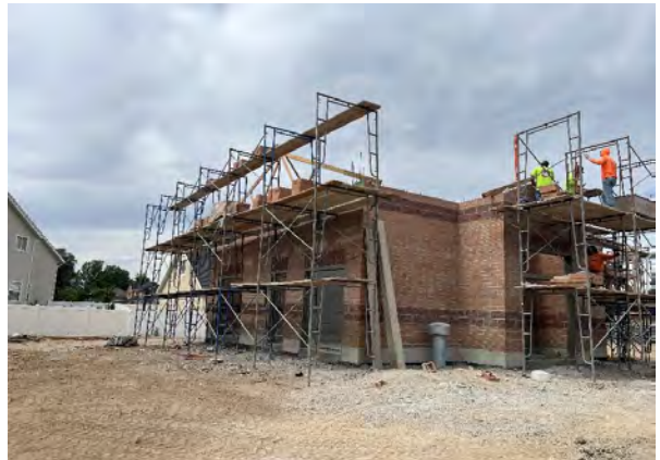
Masons installing block walls at the 1000 East site
