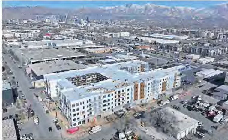
Kristin Murphy, Deseret News A luxury apartment building called The Whitney is under construction in Salt Lake City on Jan. 28. Salt Lake City is a step closer to matching a new state law requiring cities to plan for water needs in city plans.
