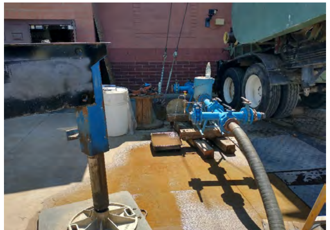
Well redevelopment sand measurement equipment
