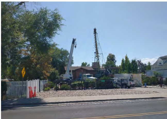
Contractor's equipment set up for well redevelopment
